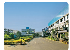
Igarashi Motors India Ltd, India
